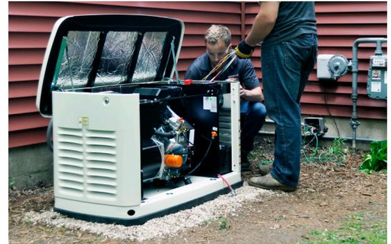
**TIP** When using plantings as a screen to hide a generator, keep the foliage trimmed at least 3 feet from the front and both ends of the box and make sure overhanging branches are at least 5 feet above the top of the box.
